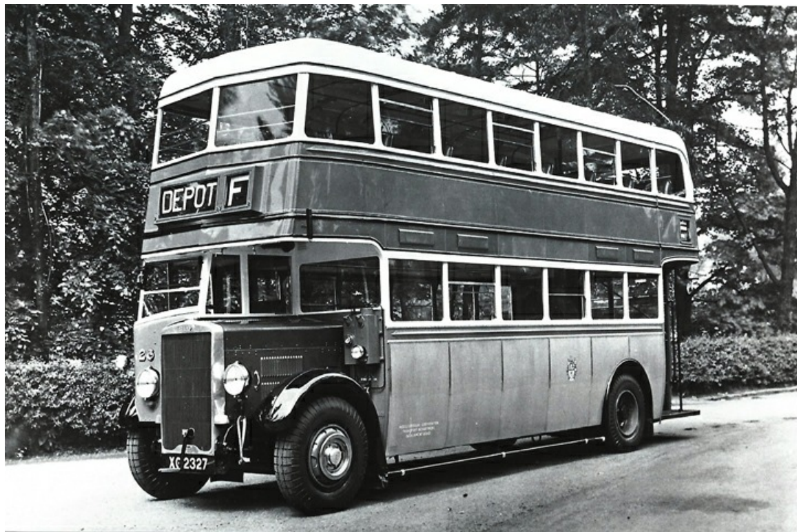
No. 26 (XG2327) was a 1934 Leyland TD3c 'Titan' with Leyland L27/24R bodywork. (Bus Archive).
