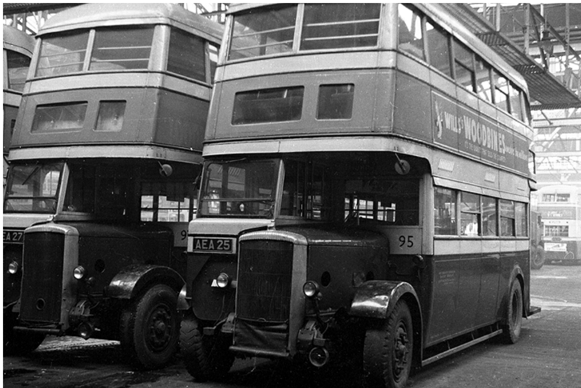
No. 95 (AEA25) was one of over thirty Daimler COG6 chassis with Metro-Cammell H30/26R bodywork acquired in 1939 for use on former tram routes. (LTHL collection).
