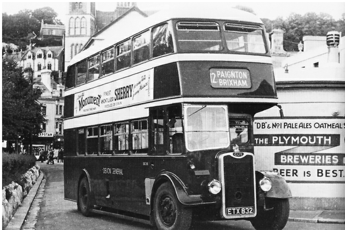
DG318 (ETX832), a 1942 Guy Arab I with Weymann 56-seat bodywork was one of two that came from the Rhondda Transport Company in exchange for two Daimler vehicles of similar age. (The Bus Archive).
