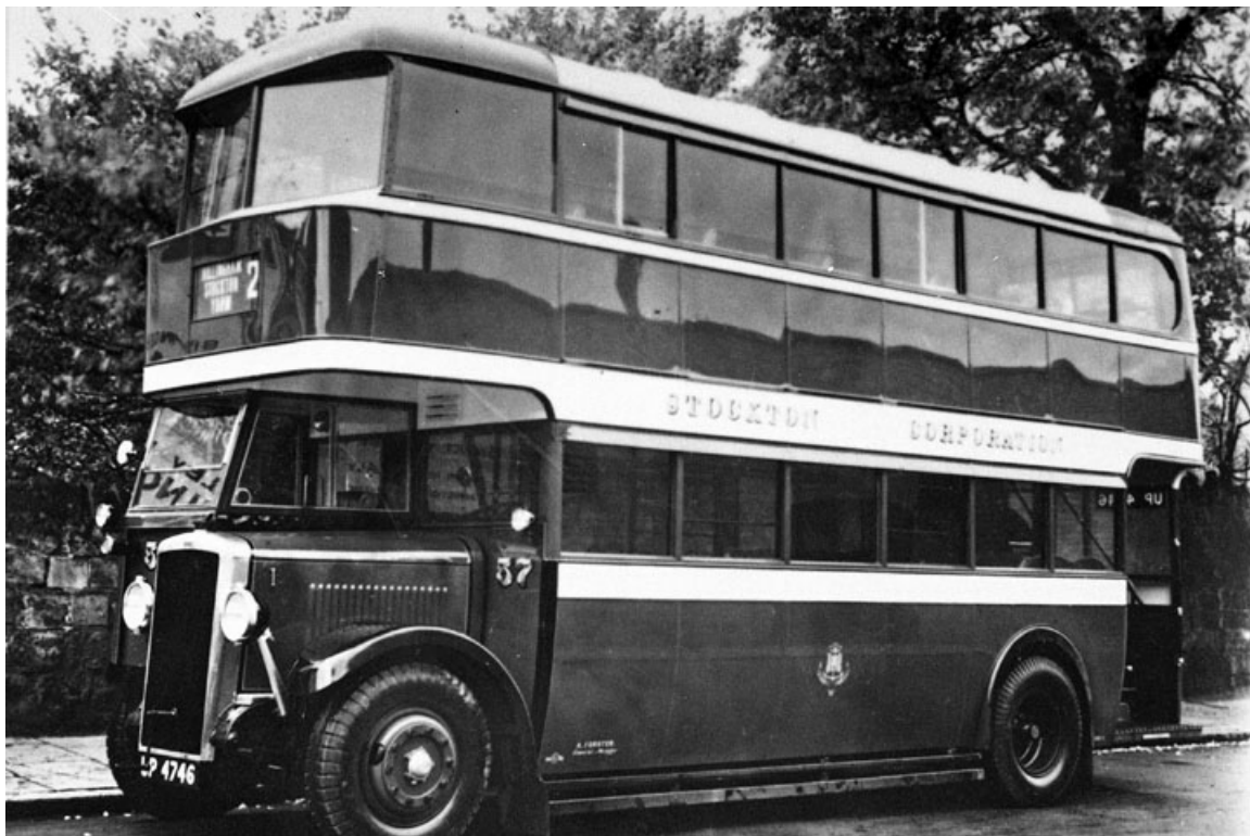
No. 57 (UP4746) was on loan from 1930. It was a Daimler CG6 with Park Royal H26/24R bodywork. (Bus Archive).
