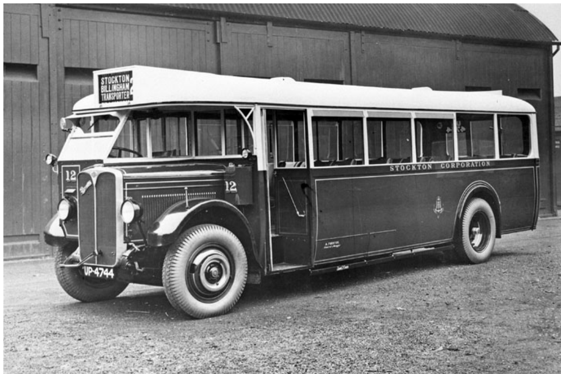
No. 12 (UP4744) was a solitary AEC Regal 4 with Brush B30F bodywork purchased in 1930. (Bus Archive).
