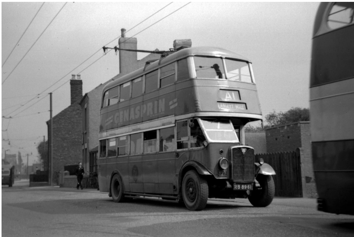
No. 327 (RB8961) was a 1933 AEC 661T trolleybus with MCCW H31/24R bodywork. (LTHL collection).
