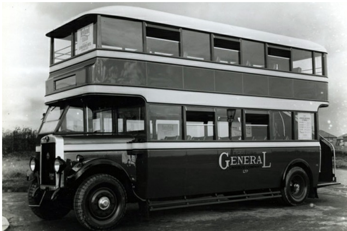
Scottish General's first double-deck vehicles were four Leyland TD1's (Nos. 201-204) with Leyland open staircase bodywork, delivered in 1929. This is one of the four when new, although its exact identity is unknown. (LTHL collection).
