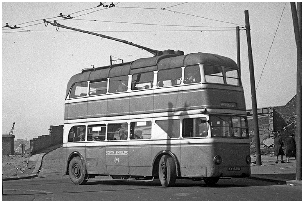
No. 235 (KY629) was an AEC 761T with English Electric H33/30F bodywork that came second-hand from Bradford Corporation in 1942. It was new in 1934 as a demonstrator. (Bus Archive).
