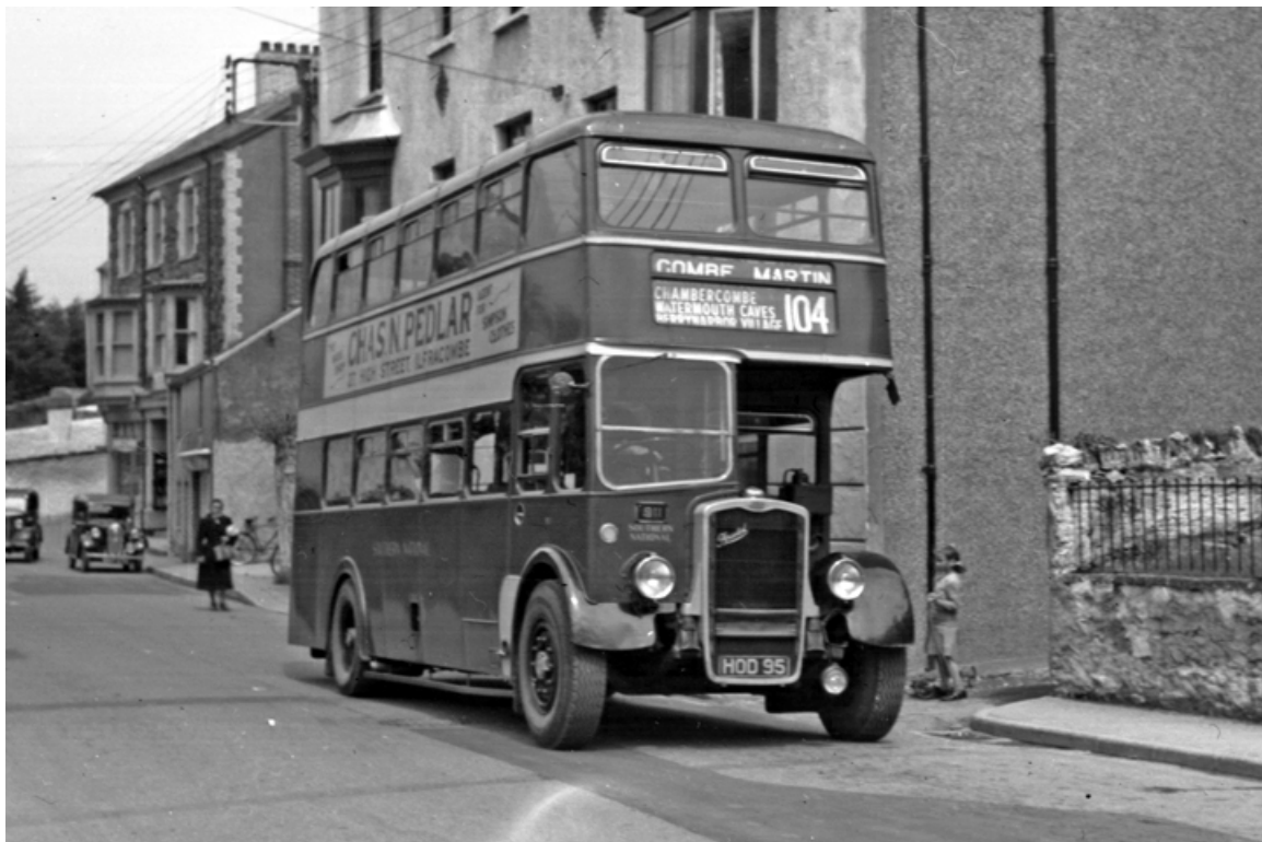
No. 911 (HOD95) en route to Combe Martin was a Bristol K5G with ECW L27/28R bodywork, new in 1949. (LTHL collection).
