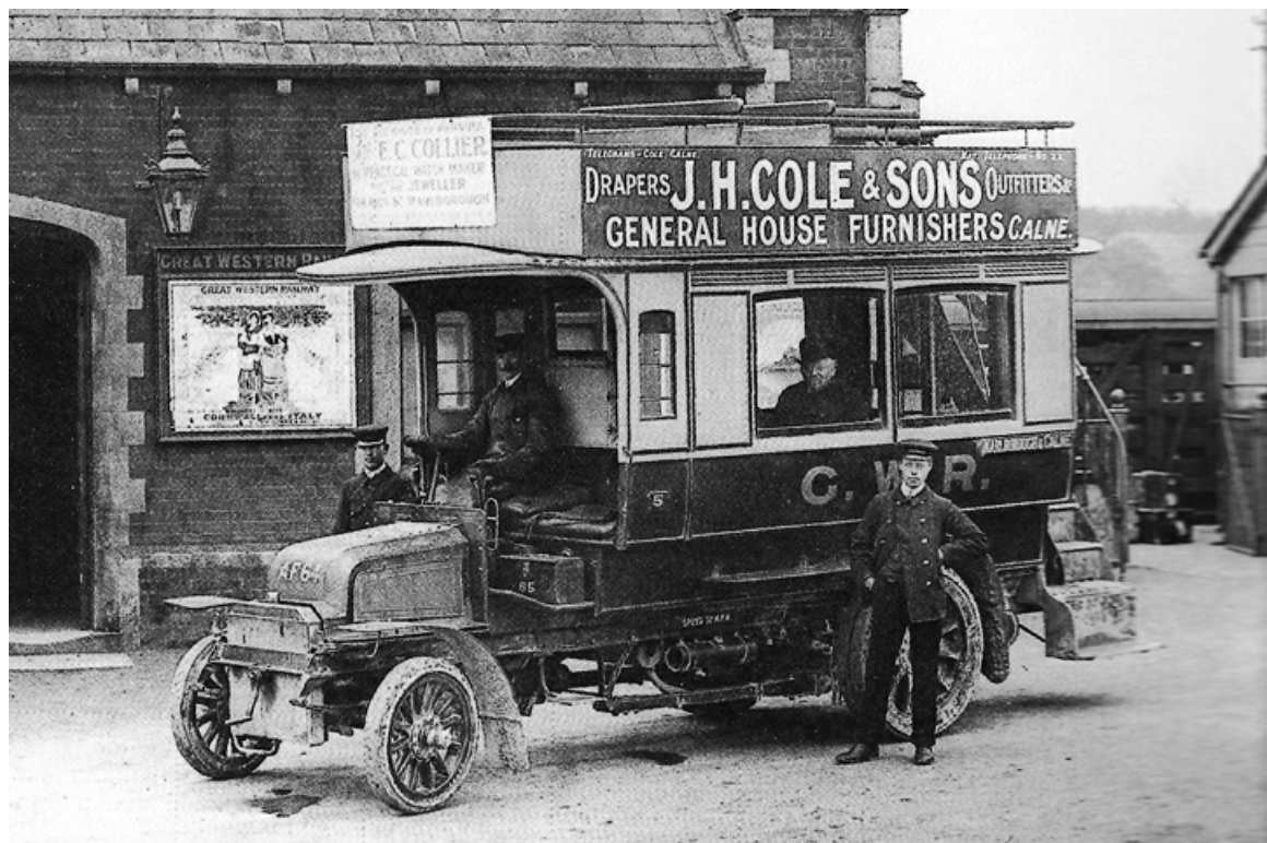
No. 5 (AF64) with 'small' double-deck 016/12R0 body. The GWR's propensity for exchanging bodies is demonstrated on page 19, which shows AF64 with a single-deck body. (LTHL collection).
