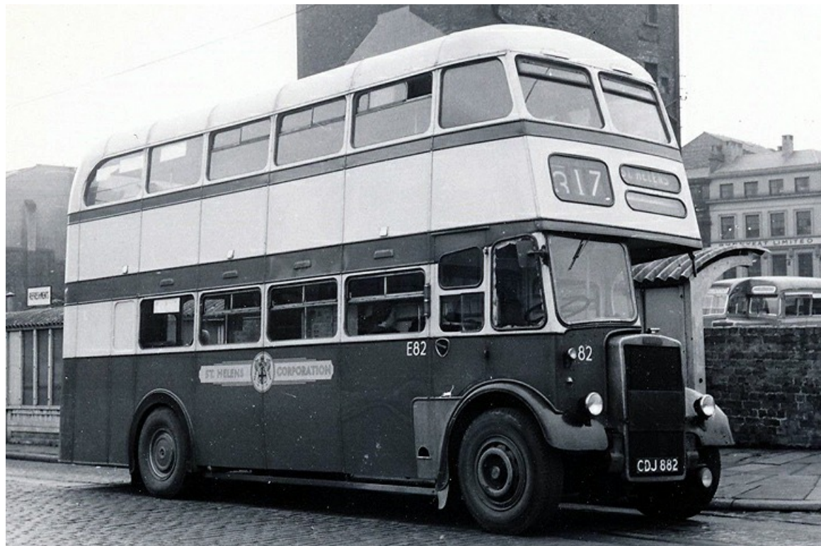
Carrying Davies 56-seat bodywork on a Leyland PD2/9 chassis is No. E82 (CDJ882) dating from 1954. (LTHL collection).
