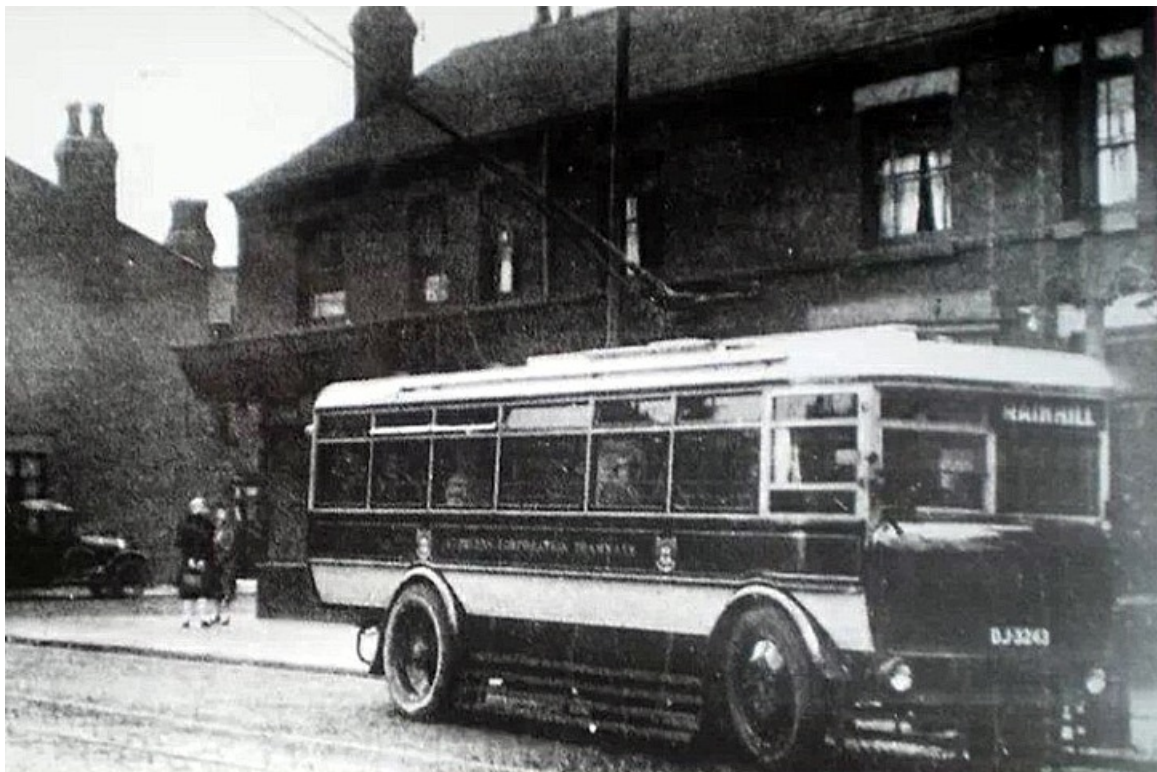
No. 1 (DJ3243) was a 1927 Garrett trolleybus with Ransomes 35-seat centre-entrance bodywork. (LTHL collection).
