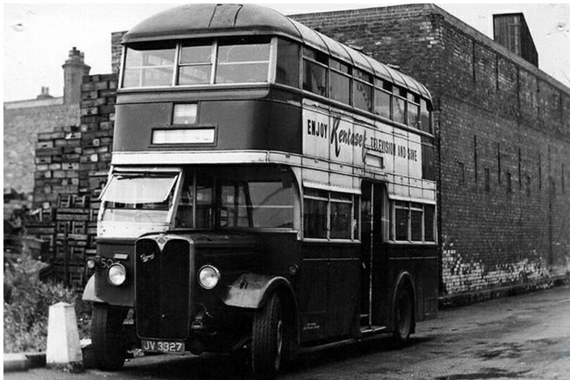
No. 50 (JV3327) was a 1935 AEC Regent with Roe 58-seat centre-entrance bodywork that was a feature of Grimsby's buses. It survived long enough to pass to Grimsby-Cleethorpes JTC in 1957. (LTHL collection).
