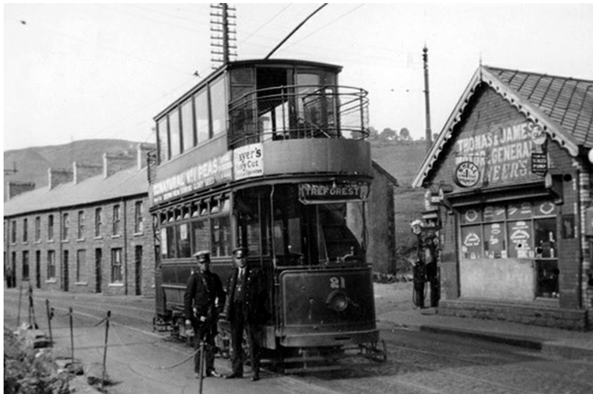
Car No. 21, a United Electric Car built double-deck tram dating from 1908, originally open top but top covered later as shown here. (LTHL collection).
