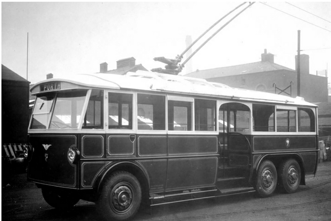
No. 7 (TG391), seen here before delivery, was an English Electric SD6WTB six-wheel single-deck trolleybus with English Electric 32-seat bodywork. (GEC collection courtesy David Beilby).
