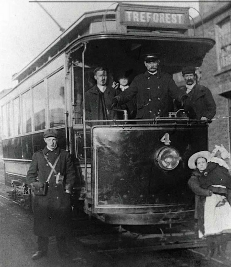
Brush-built 1905 single-deck combination bogie car No. 4. (LTHL collection).
