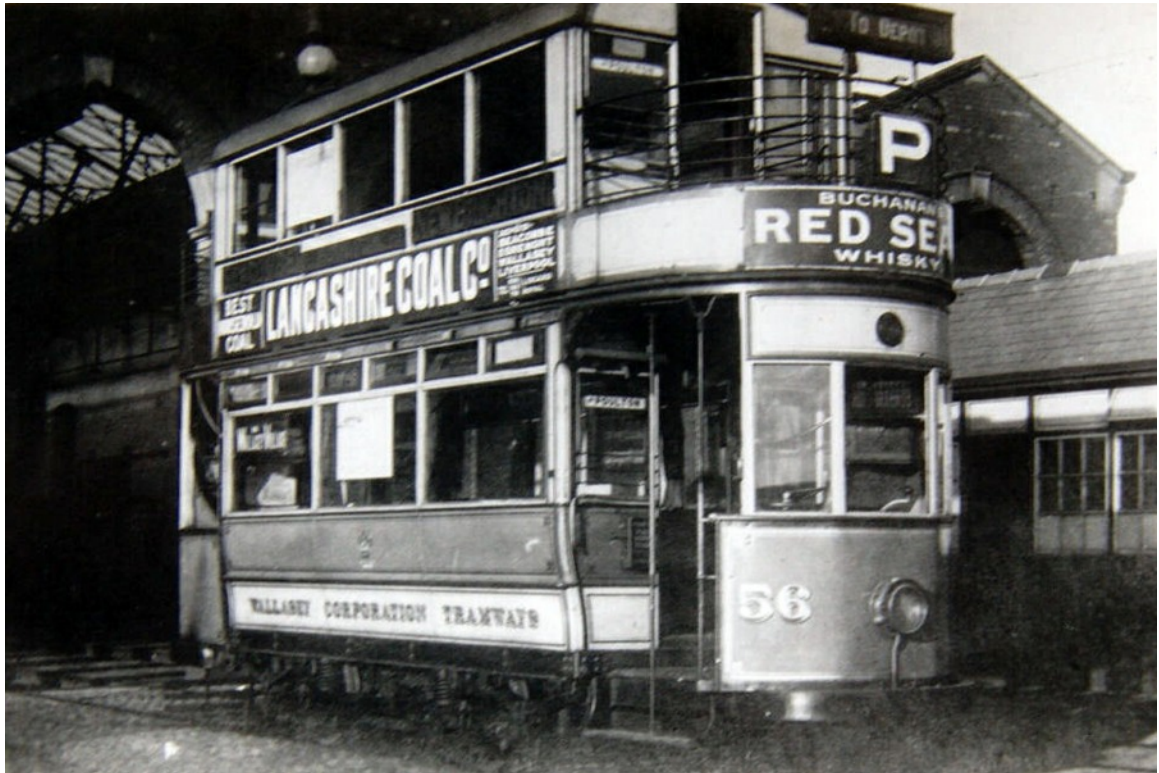
No. 56, a 1911 Brush-built top-covered double-decker on Brush trucks. It remained in service until the demise of the tramway system in 1933. (LTHL collection).
