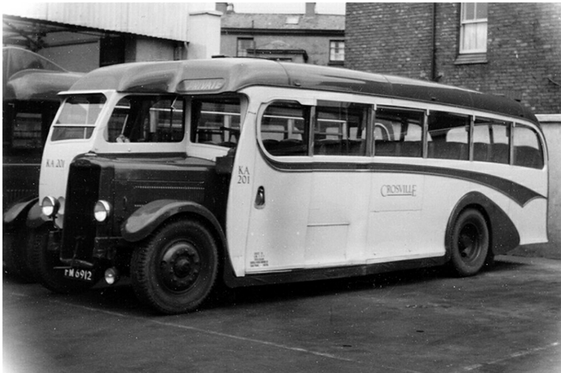
KA201(FM6912), originally numbered 641 with United B32F body, it was a 1932 Leyland TS4 re-bodied by Burlingham to C33F in 1940. It was fitted with an oil engine and re-numbered as shown in 1950. (Dennis Kerrison via Ron Hughes).
