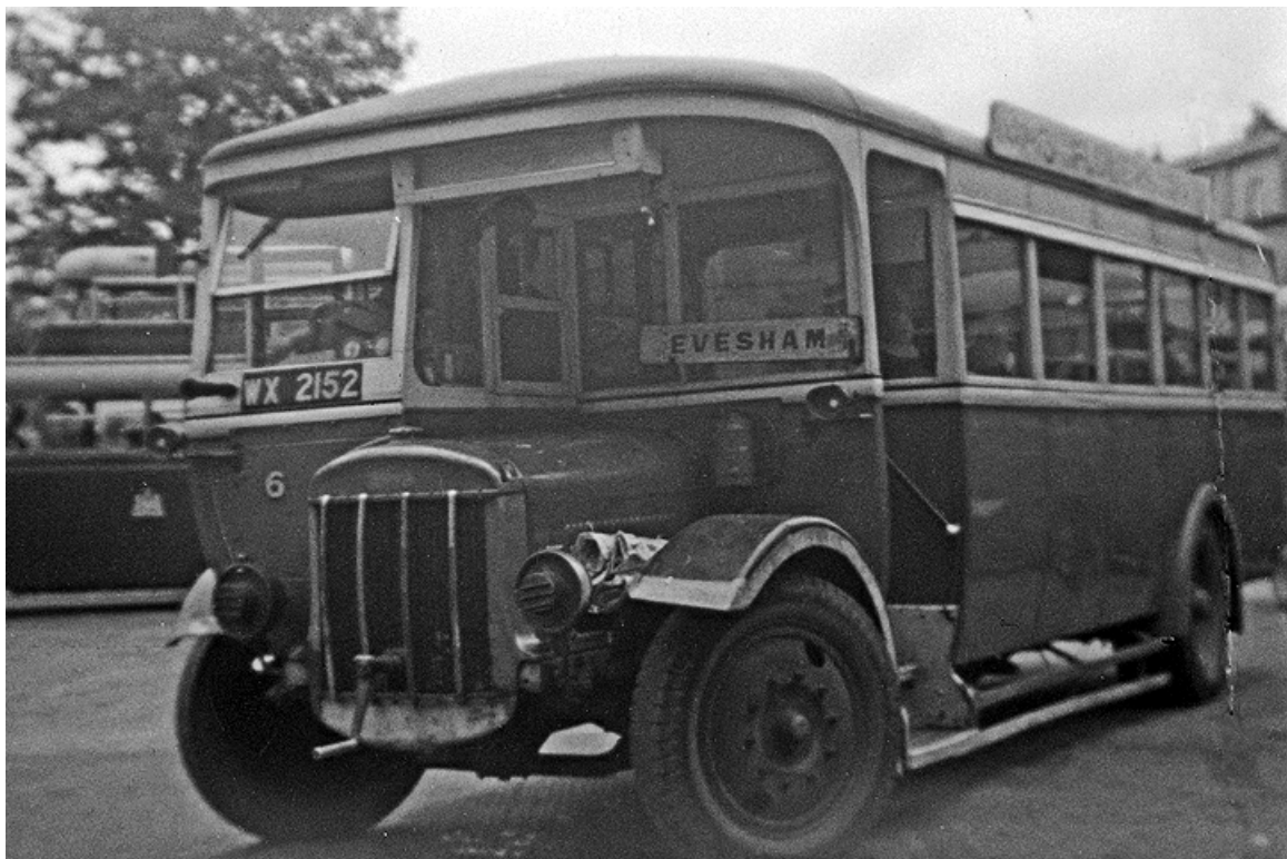
No. 6 (WX2152) was another second-hand Tilling-Stevens new in 1930, that came from West Yorkshire, this time bodied by Tilling with a B32F body. (Bus Archive).
