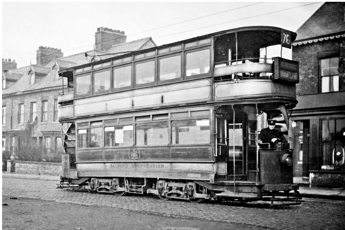
Salford No. 338 (formerly No. 109 - it was re-numbered in 1935) was a 1903 Milnes 77-seat bogie car, originally open top, it is seen here with its McHardy and Elliott top cover fitted in 1923. (M. J. O'Connor).
