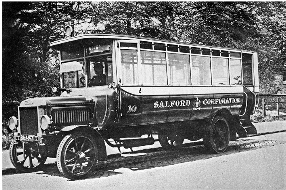
Salford's No. 10 (BA4147) was a 1923 Leyland LG1 with Leyland B32R bodywork. (Bus Archive).
