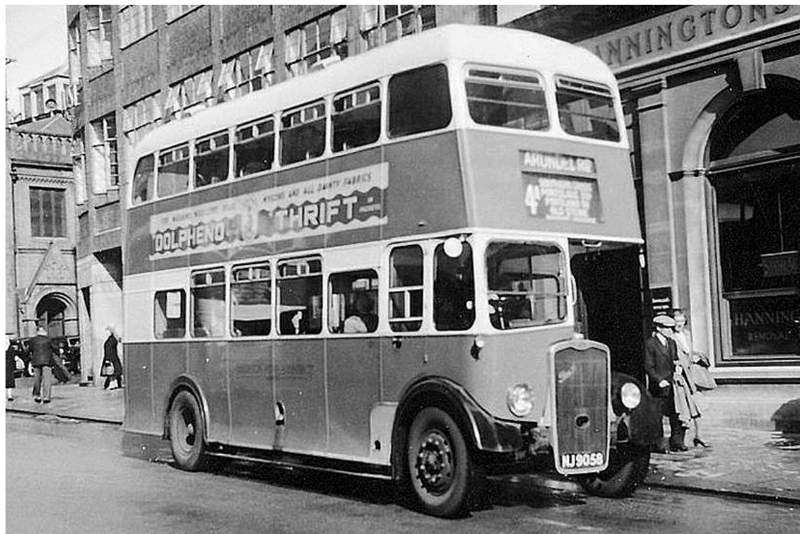
No. 6325 (NJ9058) was a 1936 Bristol GO5G originally with a Tilling 56-seat body but rebuilt by Brighton, Hove & District in 1950. It was withdrawn in 1953. (Wimborne Railway Society Archive).
