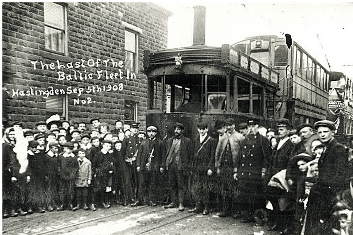
One of Haslingden's last steam trams photographed on 5 September 1908. Both loco and trailer are devoid of markings suggesting that no fleet name or numbers were used. (LTHL collection).
